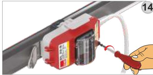
Open the transparent cover of the tap-off box by untightening the screw.
