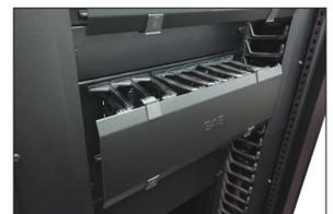
Bottom Panel : KD Server with 3 x adjustable & displaceable bottom panels and 2 x PDU cable grommets ; KD Network with 4 x adjustable & displaceable bottom panels with 2 x PDU cable grommets
