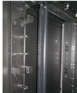
Horizontal Cable Management: metal and plastic cable organizer in different rack units, plastic finger cable troughs
