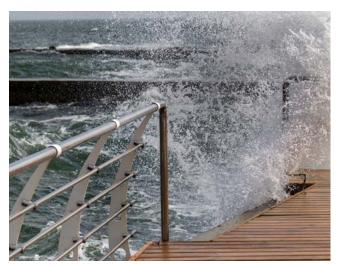
conditions according to the application area specifications. By this reason, it is not recommended to use 304 grade stainless steel in marine applications without taking special precautions. In cold climate zones, chlorides are used as defrosting chemicals and also, can cause point corrosion on 304 stainless steel surfaces.
